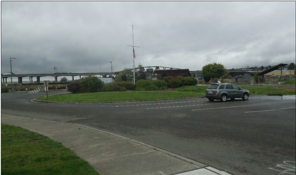
Figure 11. Overview of southern part of existing Ebey Waterfront Park, eastern half of overall project area, including turn-around, parking, and bathrooms and playground in background. View to the southwest.
