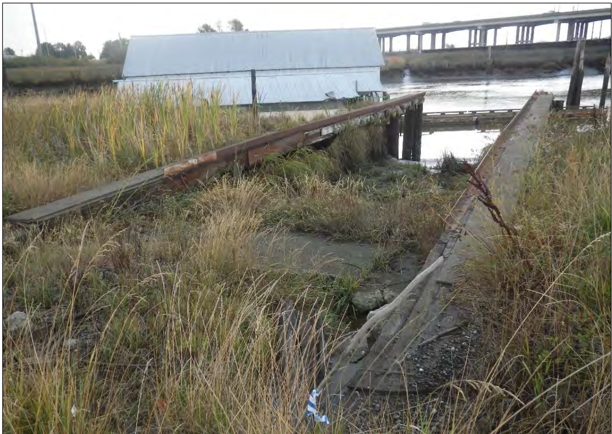
Figure 23. Boat Launch 1, extending over the Ebey Slough intertidal on pilings. View to the south.
