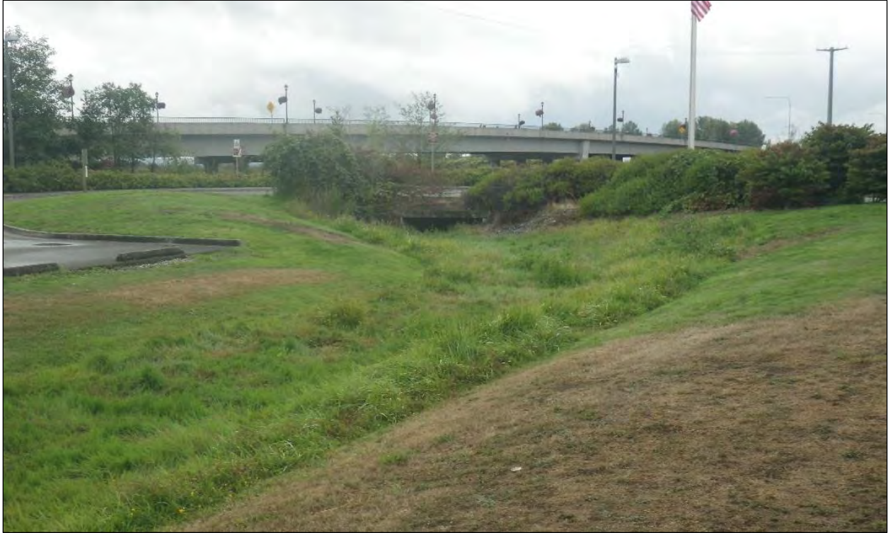
Figure 12. Artificial drainage swale and concrete culvert under access drive turn-around. SR529 Ebey Slough Bridge in background. View to the southeast.
