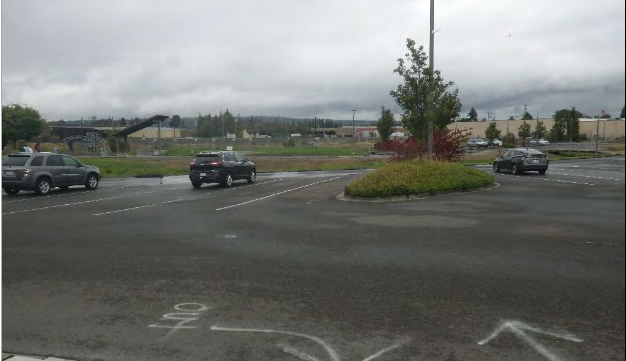
Figure 10. Overview of parking area in central portion of existing Ebey Waterfront Park, eastern half of overall project area. View to the west.
