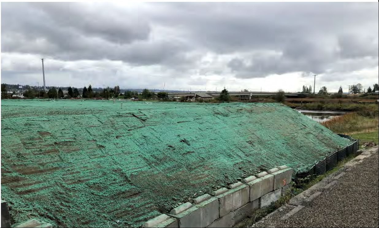
Photo 3: Preload material on Geddes Site (10/2020).
