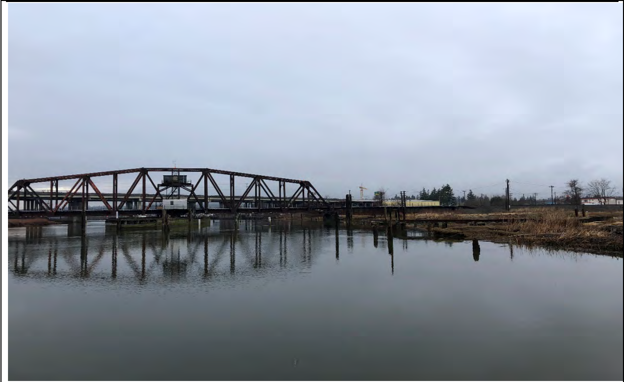
Photo 17. Photo showing that boathouses and some of the docks/floats have been removed. Old pilings still remain and will be removed as part of the expansion project (3/13/2019).
