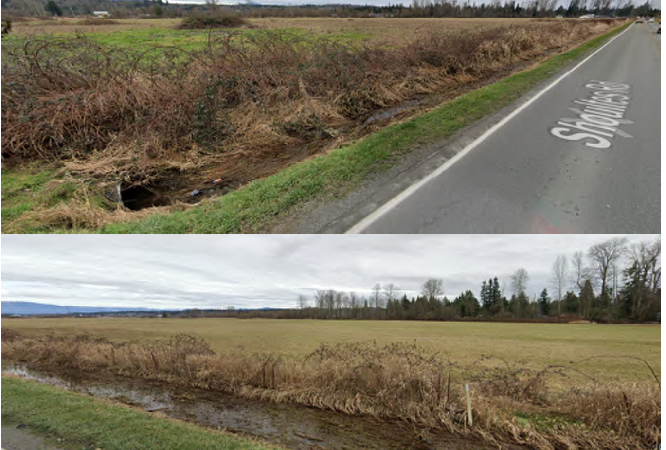
Image 2: Existing Ditch along 51 st Ave NE
