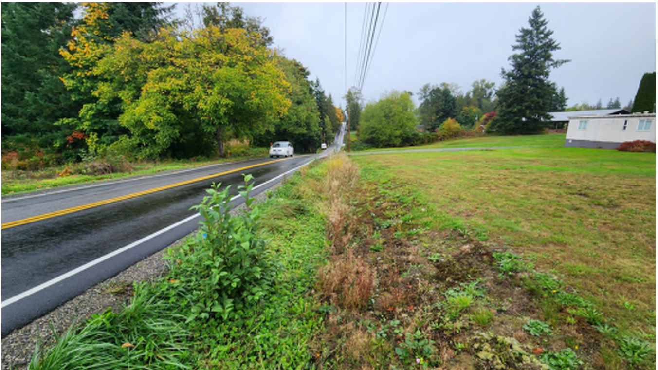
Photo 9 – Looking north along the east side of 83 rd Avenue NE at the existing ditch and culvert system that flows north.
