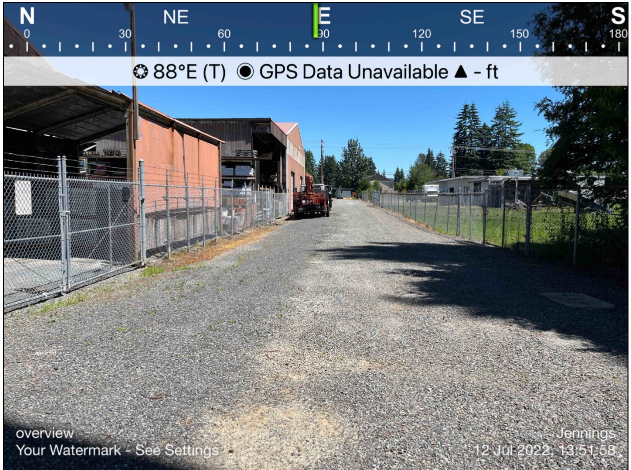
Figure 4. Overview of Gravel Driveway
