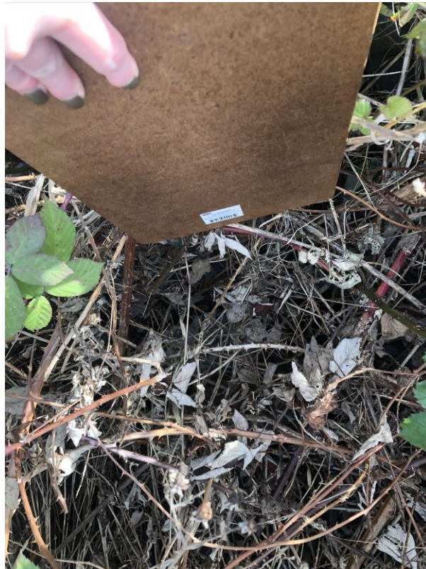
Image ④: Discharged flows are collected into an existing CMP culvert and conveyed southeastward to the existing Highway 9 collection and conveyance system.
