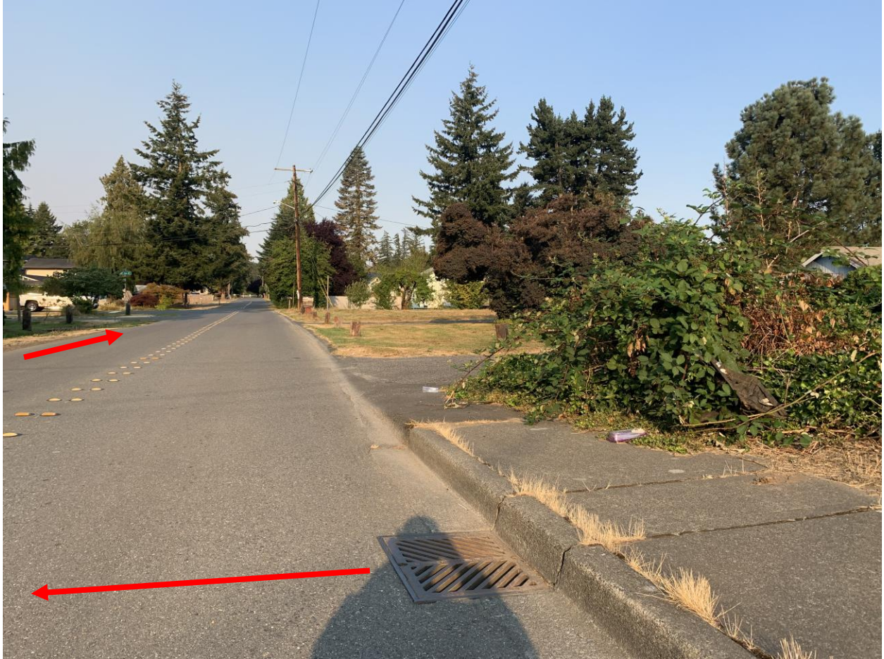
Image 4: Facing westward on 122 nd St NE near the southeast corner of the site. Stormwater runoff entering the existing City stormwater system is conveyed southward and subsequently westward along 122 nd St NE, eventually discharging to the I-5 ROW near the intersection of 122nd St NE and 35th Ave NE.
