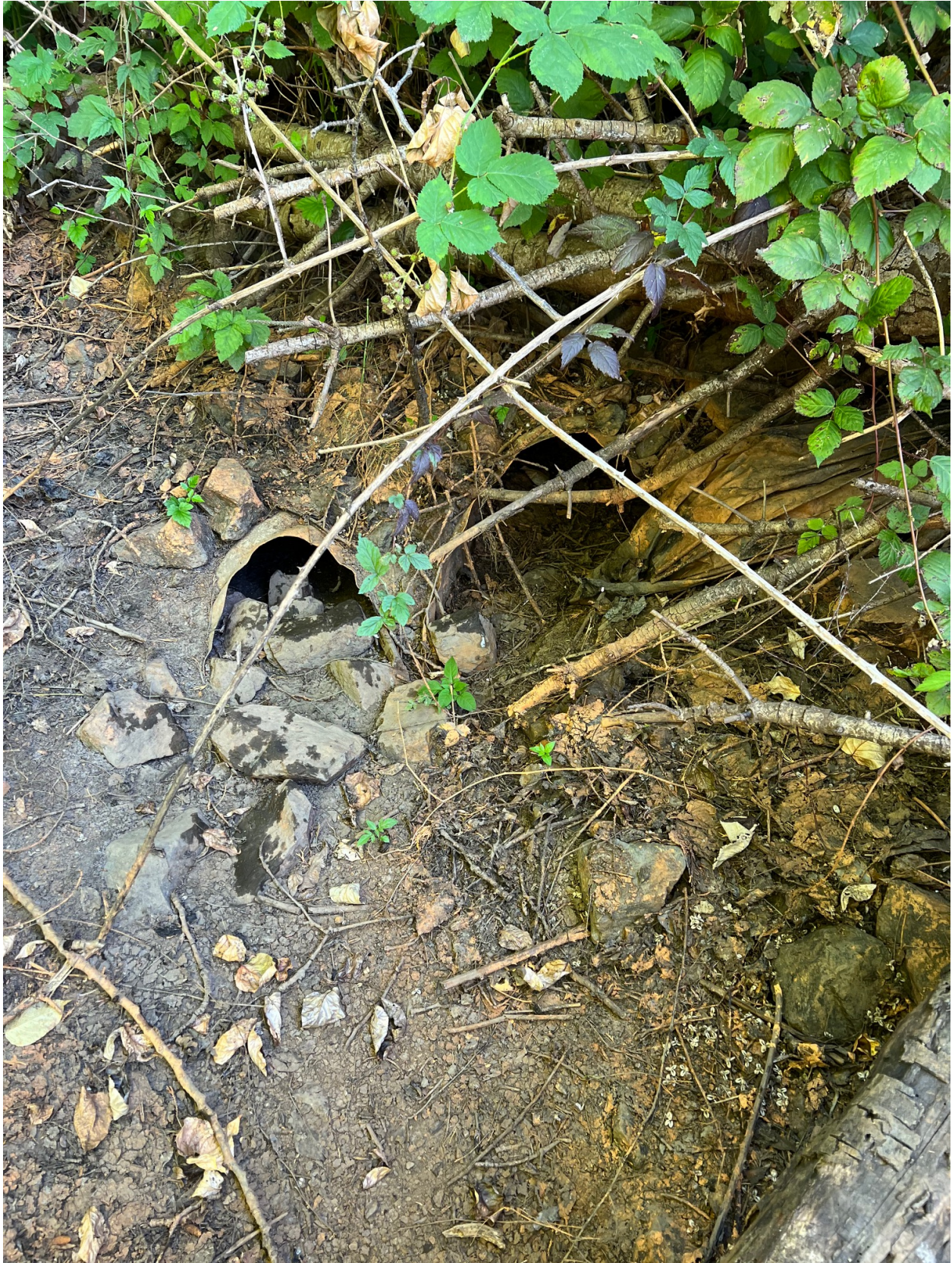
Photo 1 – Stormwater from north property
