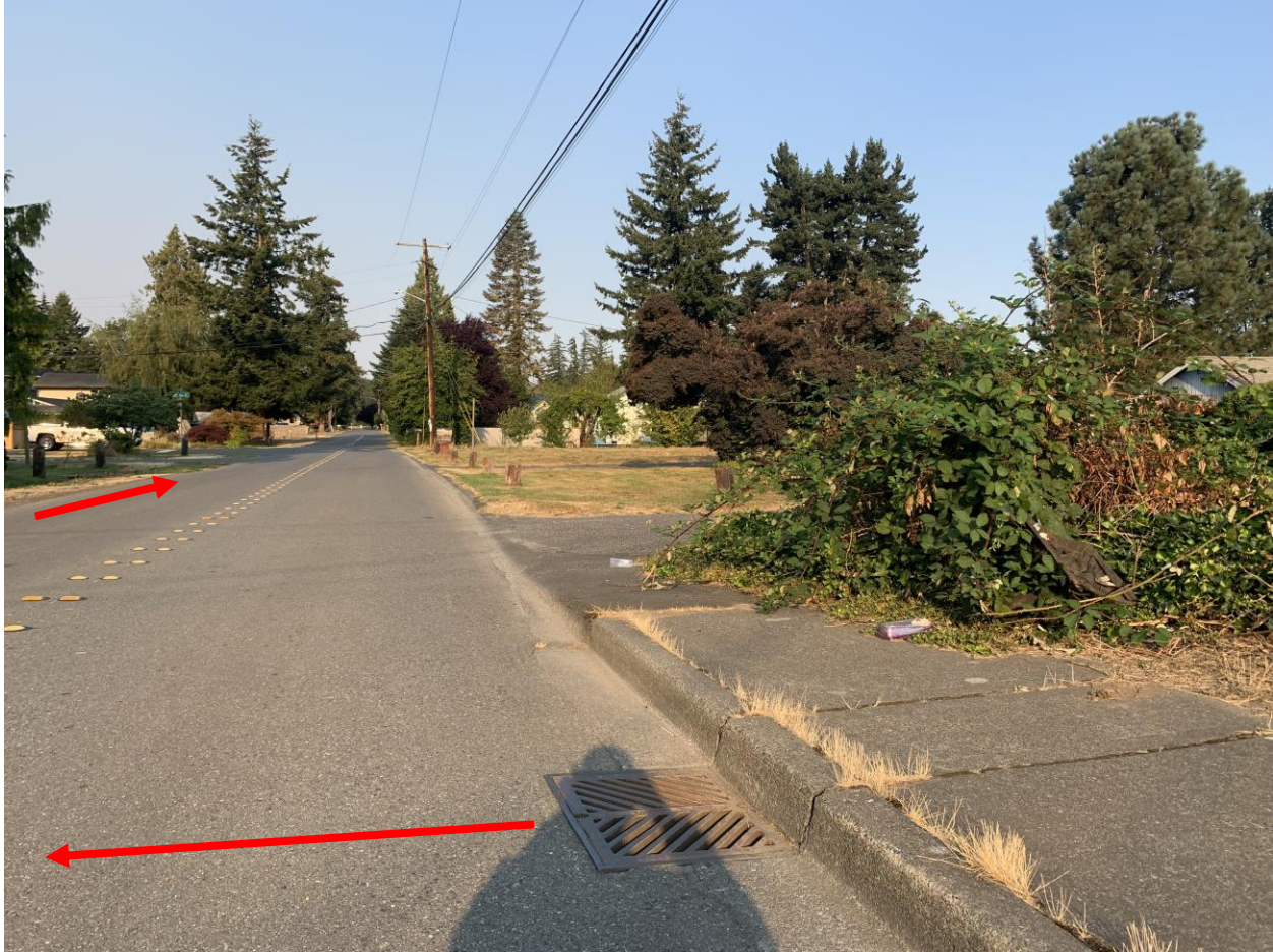
Image 4: Facing westward on 122 nd St NE near the southeast corner of the site. Stormwater runoff entering the existing City stormwater system is conveyed southward and subsequently westward along 122 nd St NE, eventually discharging to the I-5 ROW near the intersection of 122nd St NE and 35th Ave NE.
