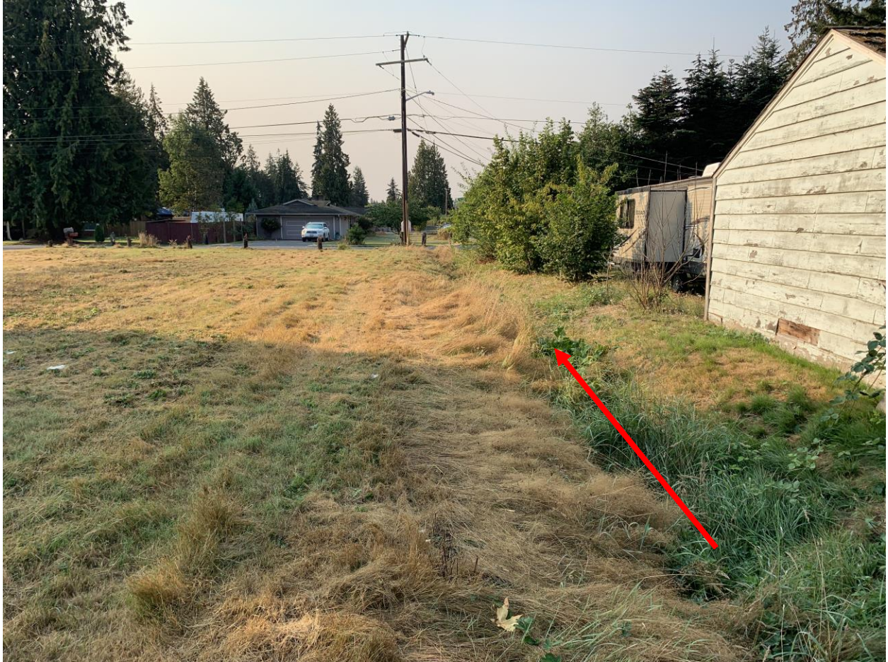
Image 2: Facing southward towards 122nd St NE along the western edge of the property. Site runoff flowing westward into the swale is directed southward, where it enters the existing City of Marysville conveyance system via a 12” culvert at the southwestern corner of the property, along the northern margin of 122nd St NE.
