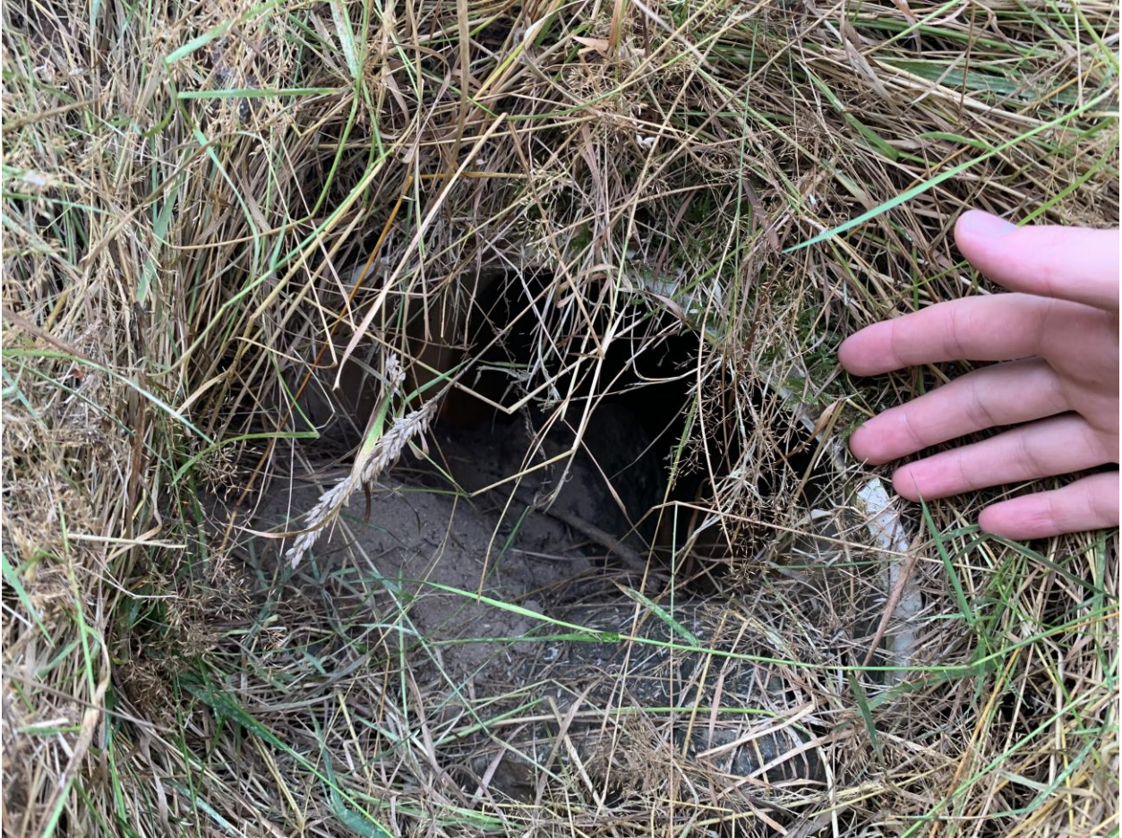
Image 3: Flow within the existing onsite drainage swale enters a 12” culvert near the southwestern corner of the property. Flow crosses southward beneath 122nd St NE before continuing westward in the existing City of Marysville stormwater conveyance system along the southern margin of 122nd St NE.
