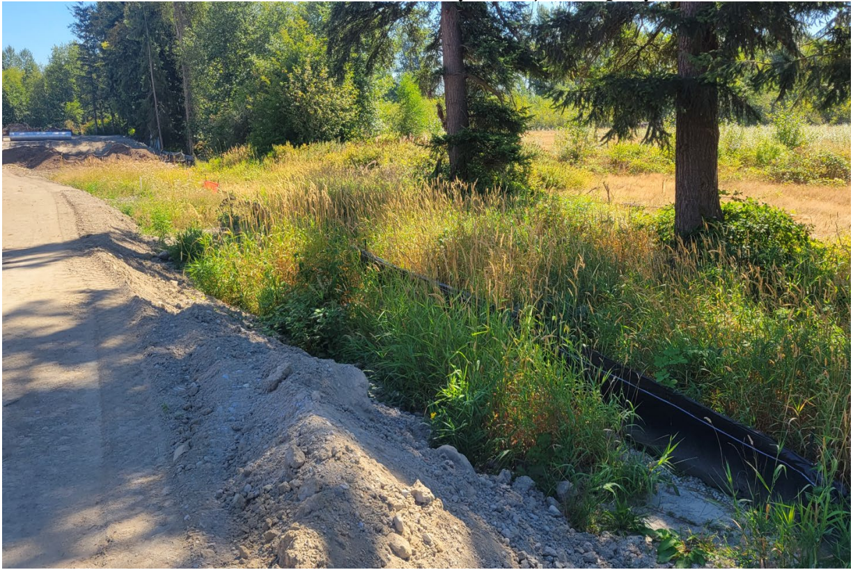
Ditch on Southern Boundary of Subject Property
