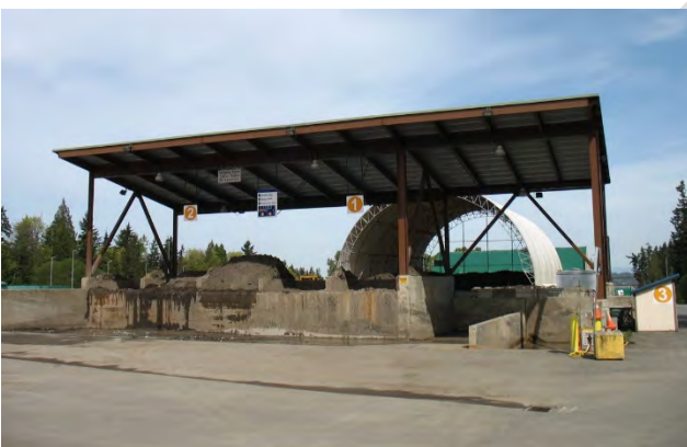
Vactor Decant Waste Facility at Cathcart
