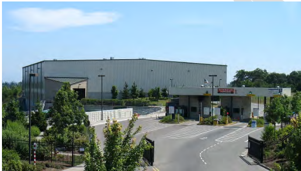
Airport Road Recycling and Transfer Station
