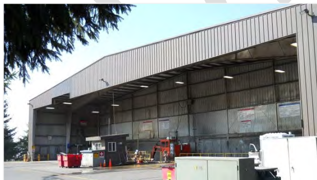
North County Recycling and Transfer Station
