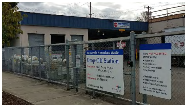
Moderate Risk Waste Facility
