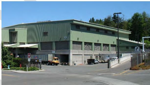
Southwest Recycling and Transfer Station
