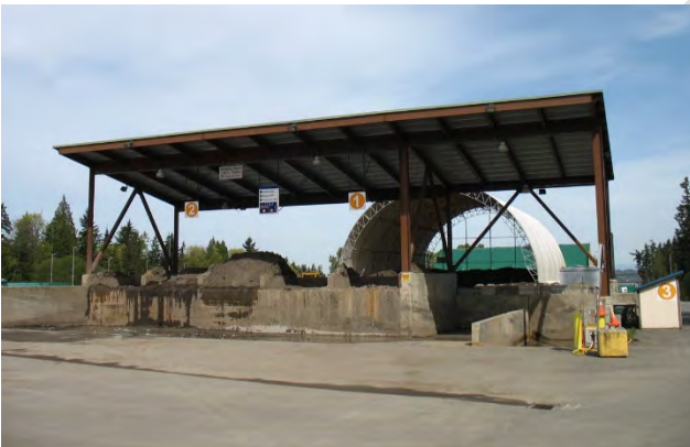
Vactor Decant Waste Facility at Cathcart
