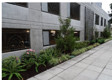
Parking garage with window openings
