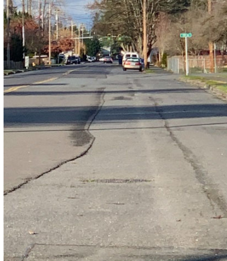
Figure 32. Quinn Ave north of 4th St
