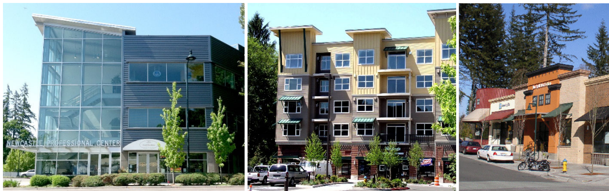
Figure 10. L-R: office building in Newcastle, WA; residential/retail vertical mixed use; stores in Mill Creek, WA
