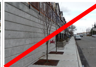
Parking garage without window openings
