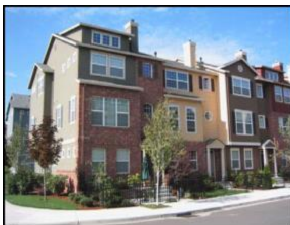
Figure 13 – This building uses brick for more than 10 percent of the facade, a decorative mix of materials and colors, decorative entries, and decorative windows to add visual interest.
