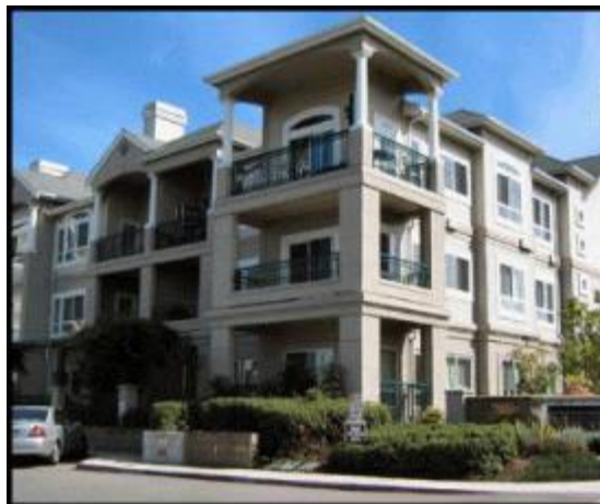
Figure B19– Balconies provide private, usable open space for residents.
