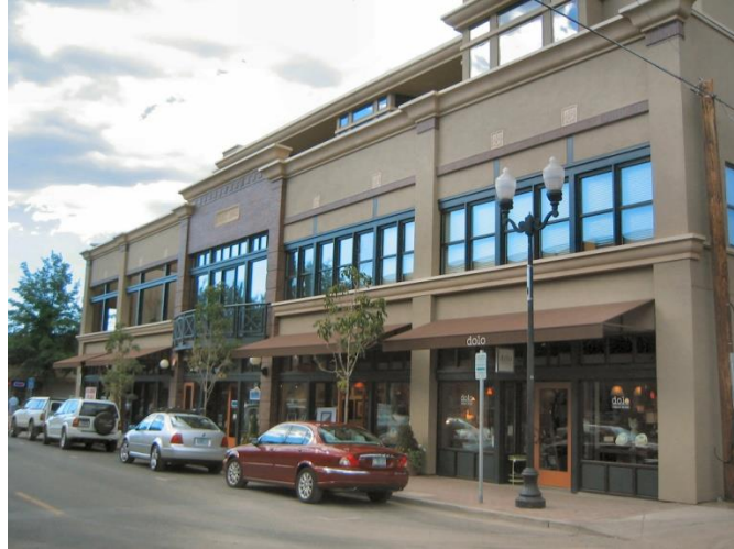
Figure C11. Example of a well-articulated building. Note how the awnings, window divisions, pilasters columns and cornice line all serve to divide up the façade into smaller segments without disrupting the unity of the overall design.
