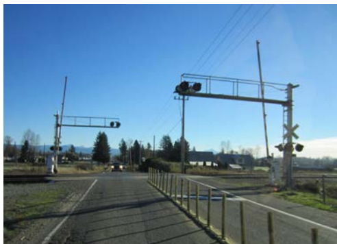
Figure 3. The railroad crossing on 172 nd Street NE delays traffic.
