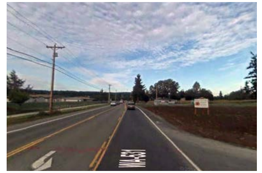
Figure 29. Existing conditions on 172 nd Street NE between 16th Drive NE and 11th Ave NE.
