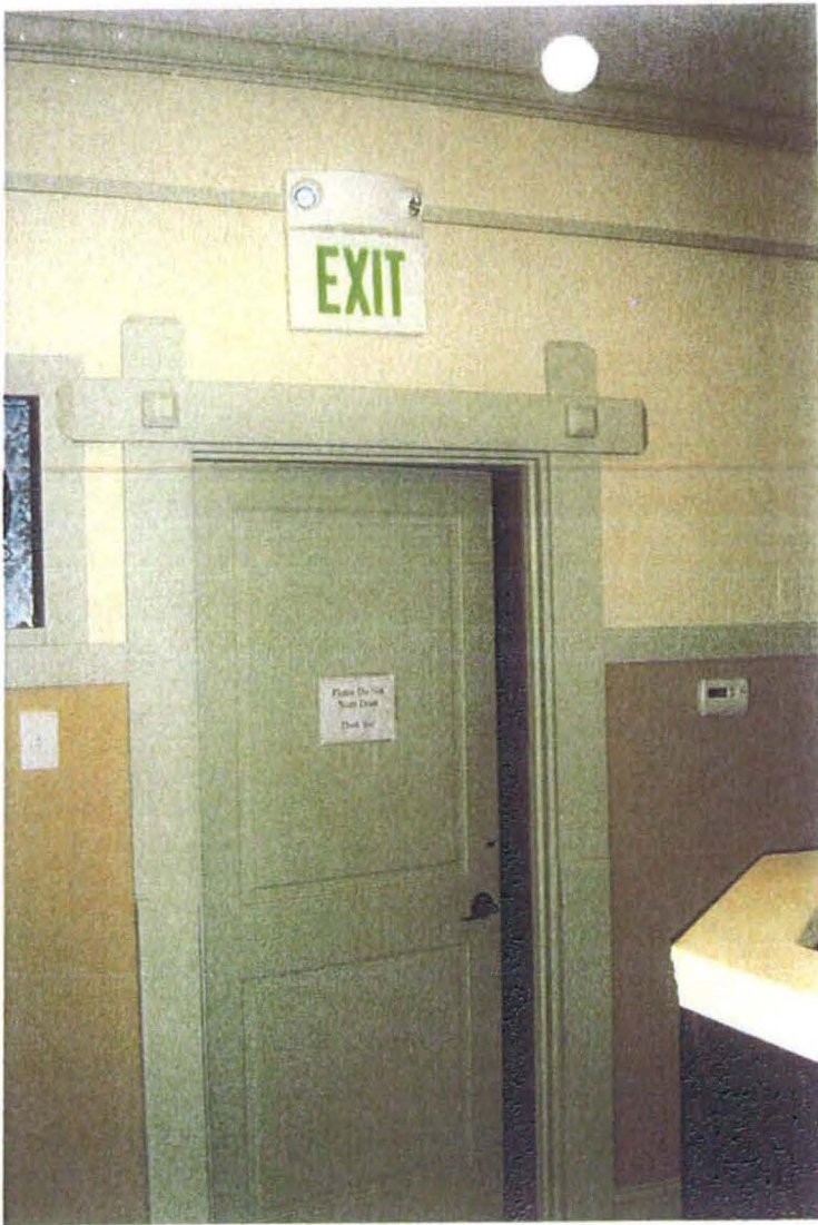
NORTH EXIT ROOM 3
