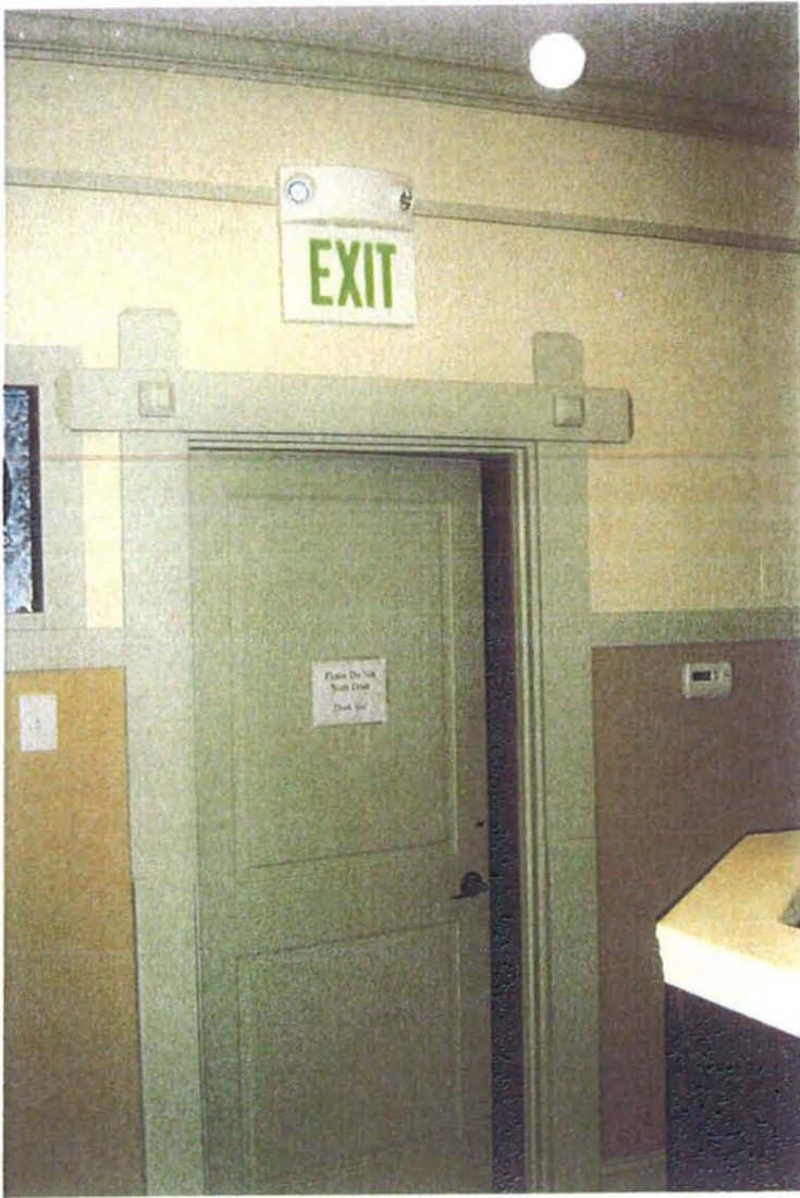
NORTH EXIT ROOM 3
