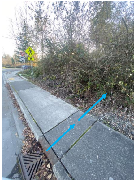
Image 8: Storm systems outlets to vegetated area at 83 rd Ave – Soper Hill intersection
