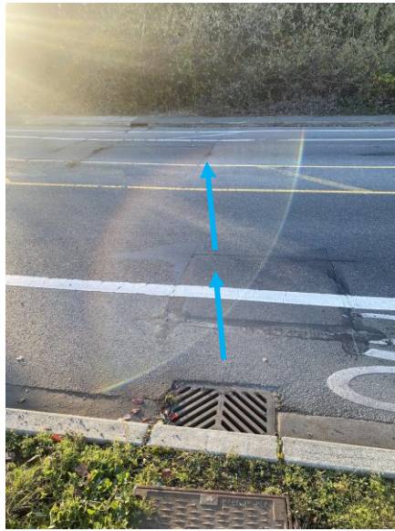
Image 7: Conveyance system crosses west under 83 rd Ave prior to Soper Hill Rd intersection
