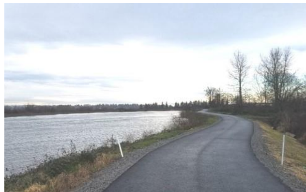
Figure 42. Newly constructed waterfront trail along Ebey Slough
