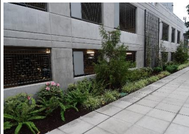
Parking garage with window openings
