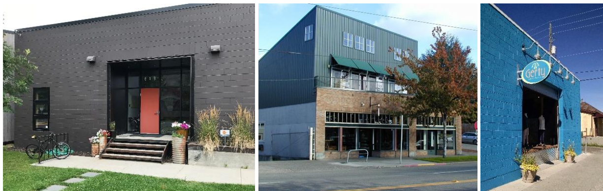
Figure 12. L-R: flexible building in Bozeman, MT; small retail/office building in Seattle, WA; retail shop in converted industrial building in Bozeman, MT
