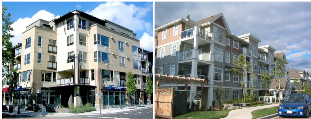
Figure 14.L-R: “four over one” mid-rise apartment building with ground floor shop; four-story apartment building
