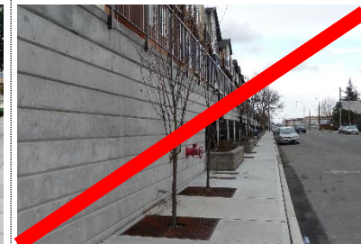
Parking garage without window openings
