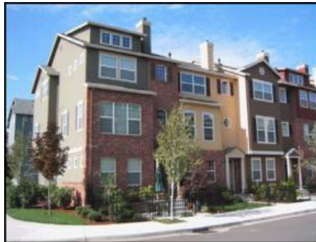
Figure 15 – This building uses brick for more than 10 percent of the facade, a decorative mix of materials and colors, decorative entries, and decorative windows to add visual interest.
