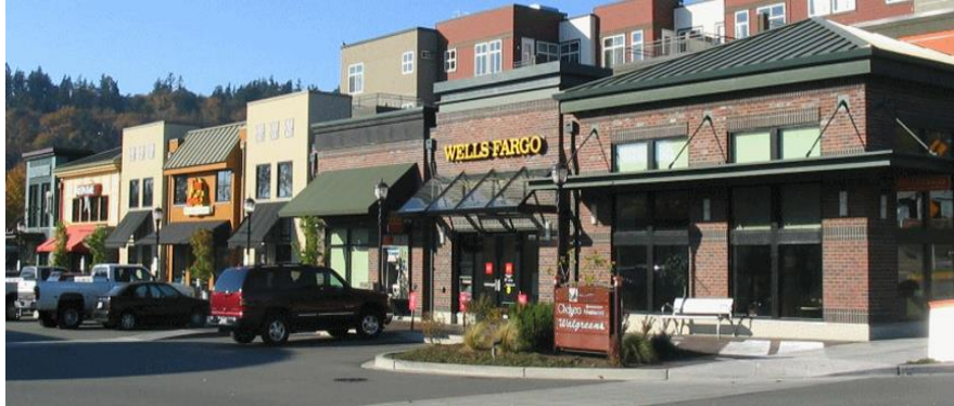
Figure 37 – This development uses a variety of roof forms, heights, and variations in roof textures by using metal hip roofs, different weather protection features, changing building materials and colors, and a modest amount of horizontal building modulation to reduce the overall architectural scale into smaller “storefront” components.
