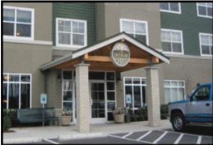
Figure 46 – A distinct, weather-protected primary building entrance.
