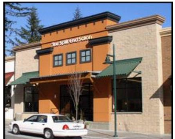
Figure 43 – This storefront effectively combines EIFS and concrete block with wood trim and metal detailing
