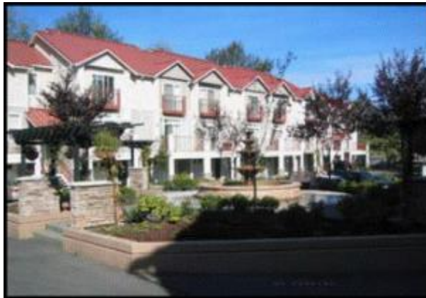
Figure 19 18 – These townhouses provide balconies and semi-private yard space.
