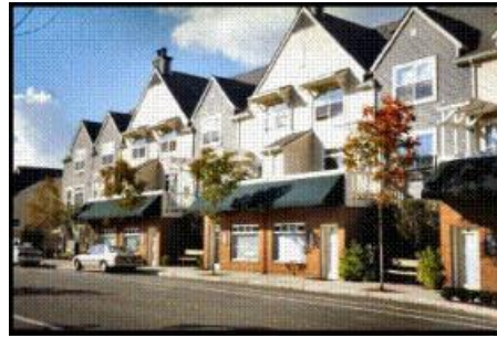
Figure 33 – Illustrating a variety of human-scale components on a building.
