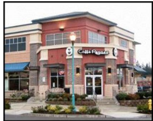
Figure 40 – Decorative use of windows, change of materials, and special lighting create a statement at this corner location.
