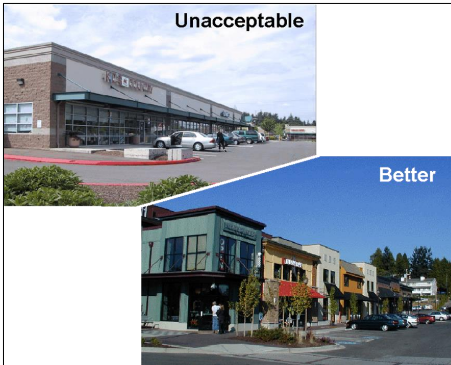
Figure 31 – The continuous canopy on top is monotonous and deemphasizes individual storefronts. The bottom example provides a variety of weather protection features and represents a more desirable example
